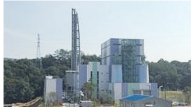
Jungbu Electric Power Co., Ltd.
